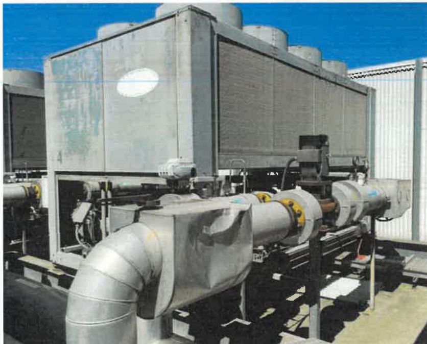
Typical - Air Cooled Chiller Primary including Flow / Return pipework, Valves and Circulation Pump
