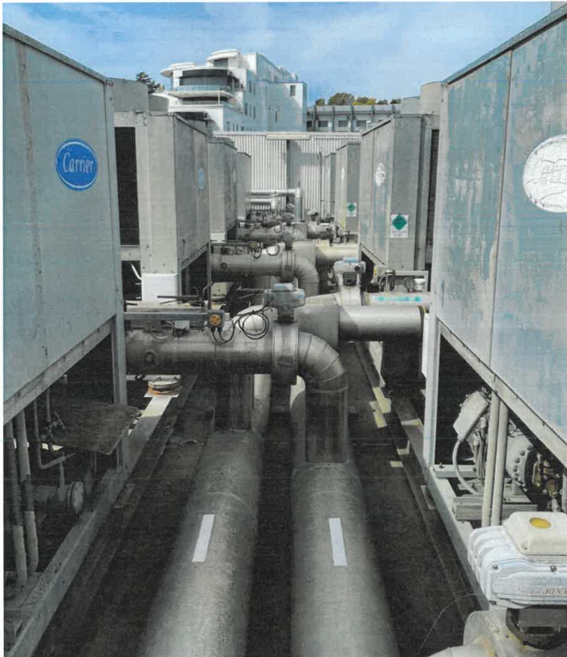
Primary Flow / Return pipework Headers at ground level with connection to all Air Cooled Chillers
