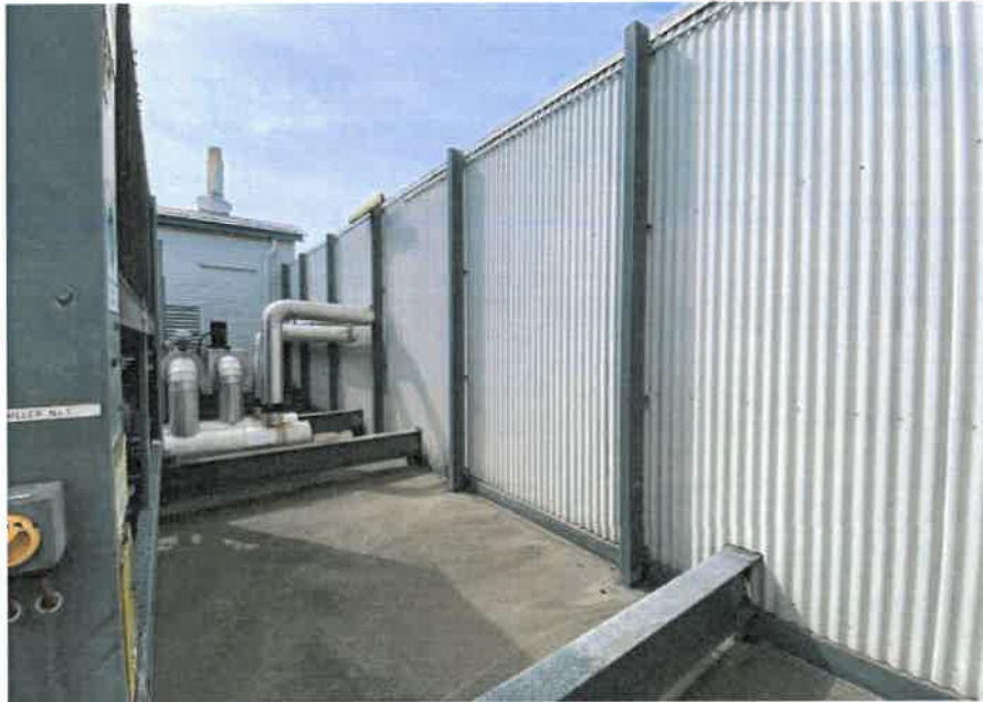
Example of solid acoustic walls around 3 sides of the plant area with the boiler house at one end
