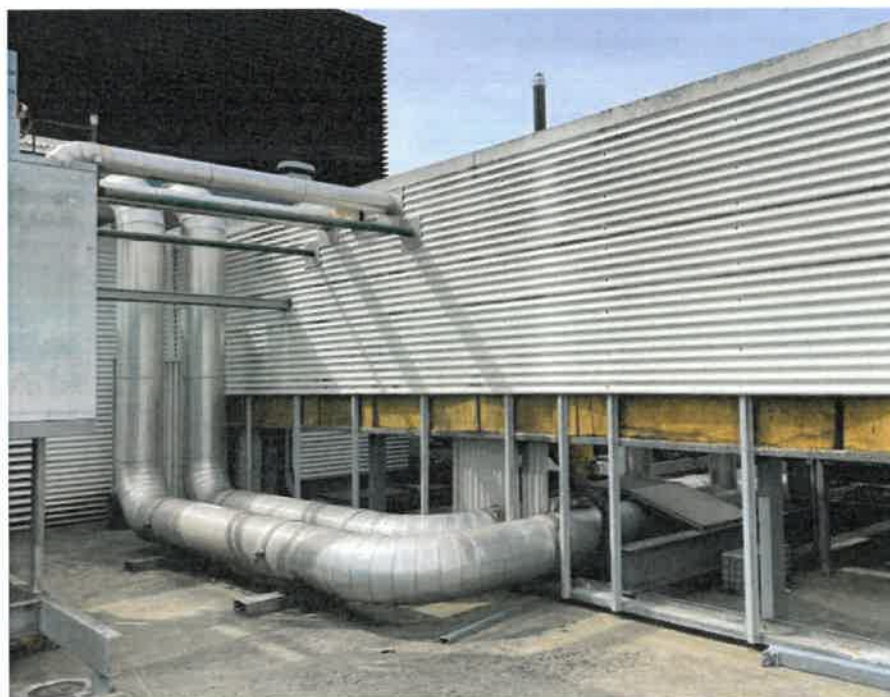
Primary Flow / Return pipework Headers to building (note: partly removed solid acoustic wall at one end of plant area to improve airflow)
