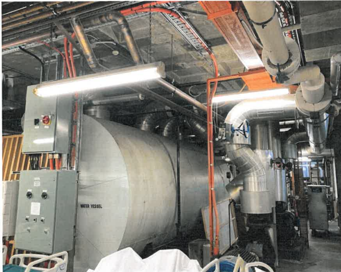
Chilled Water Vessel, Secondary Circulation Pumps and associated VSD's and Switchboards
