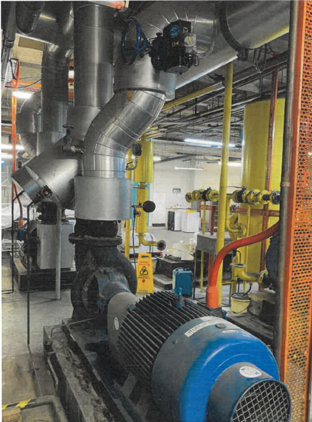
Chilled Water Secondary Circulation Pumps
